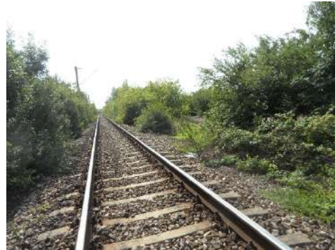
Zona tunel km ex.7+931
