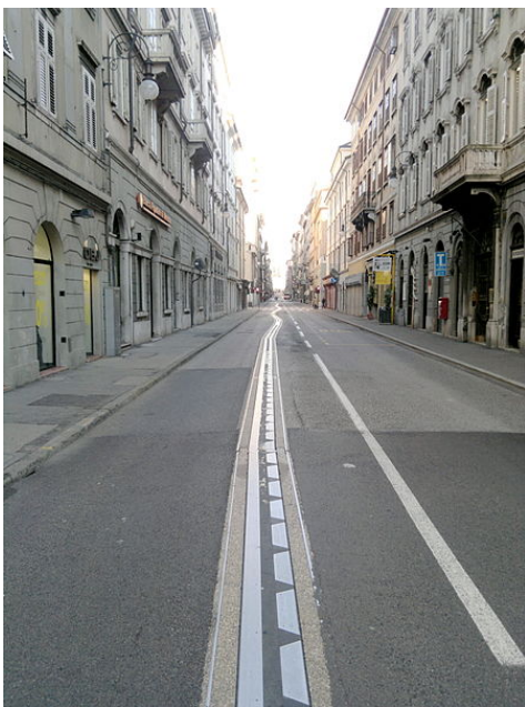
Fig.: Conductor rail for the “Stream” system in Trieste (source: wikipedia)
